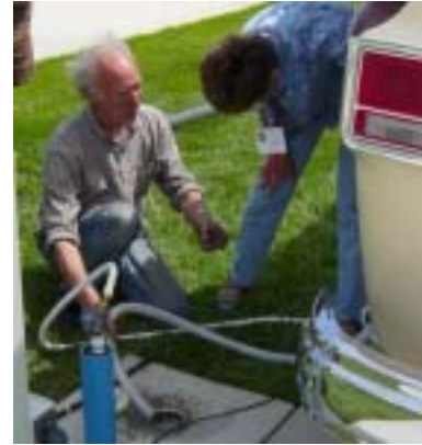
Denny Allen Installing Macerator
